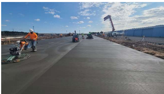
Figure 3- Finish work on the foundation slab
