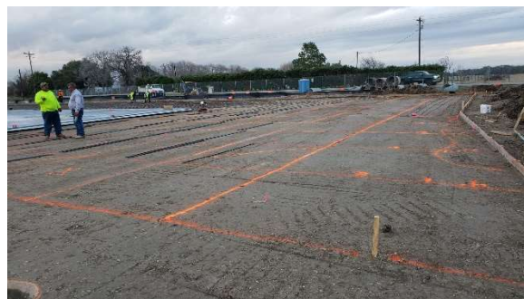
Figure 4 – Layout for the apron pavement
