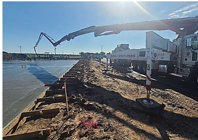
Figure 2 – Concrete placement of the foundation
