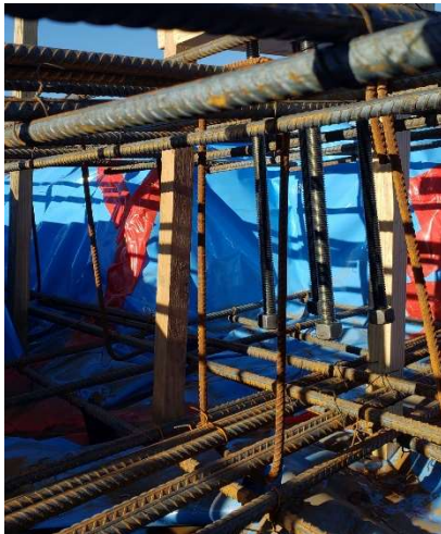
Figure 1- Reinforcing steel in building foundation
